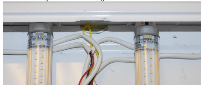
Figure 8: Example of wire routing in recessed luminaire
