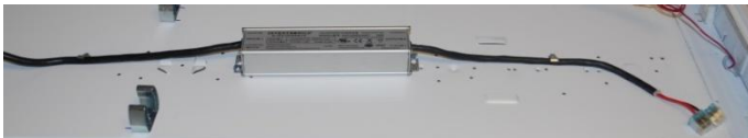
Figure 1: Example for an installed LED Driver in the wire way of a recessed luminaire.
