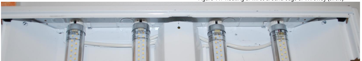
Figure 12: Completed installation of Wireway.
